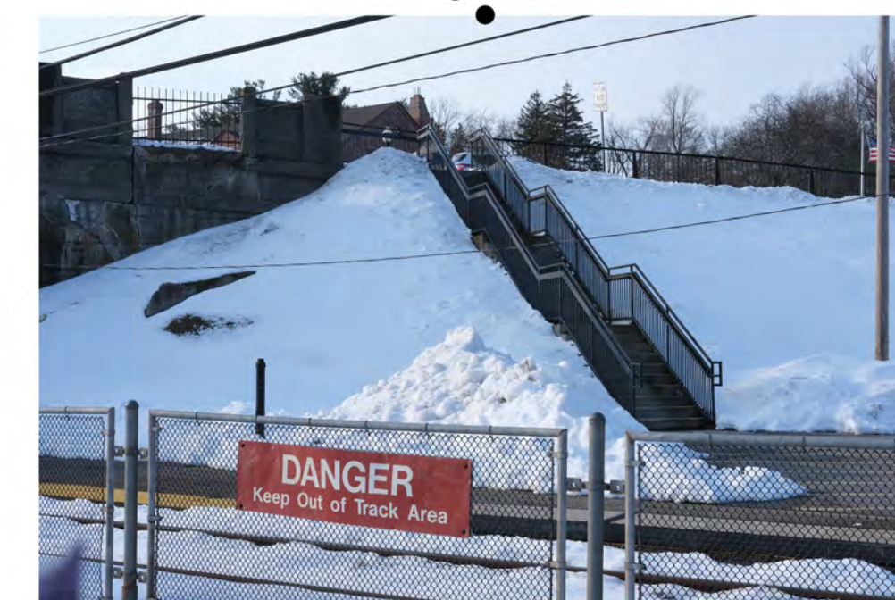
Steep Slopes at Noble Station
