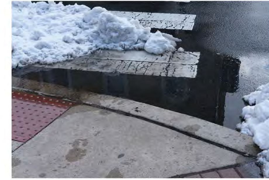
Water collecting on impervious sidewalk and road
