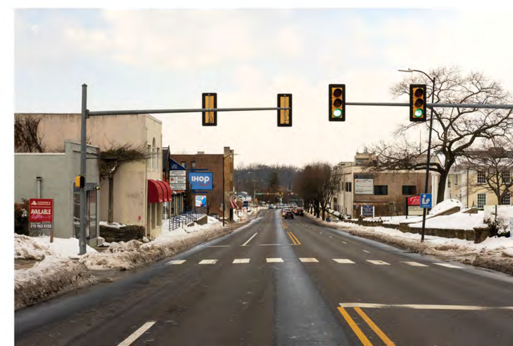
Old York Road Looking North
