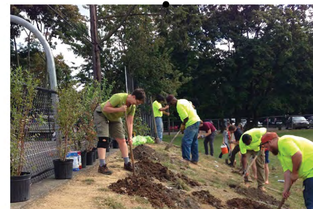
Steep Slopes at Jenkintown High School
